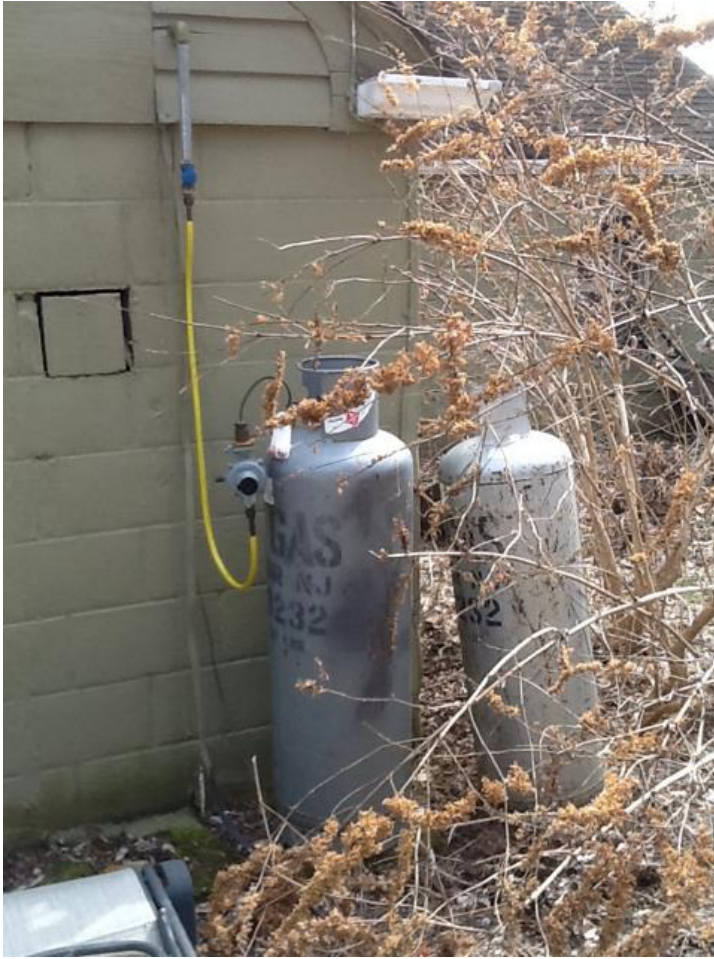
Propane tank at exterior above grade
