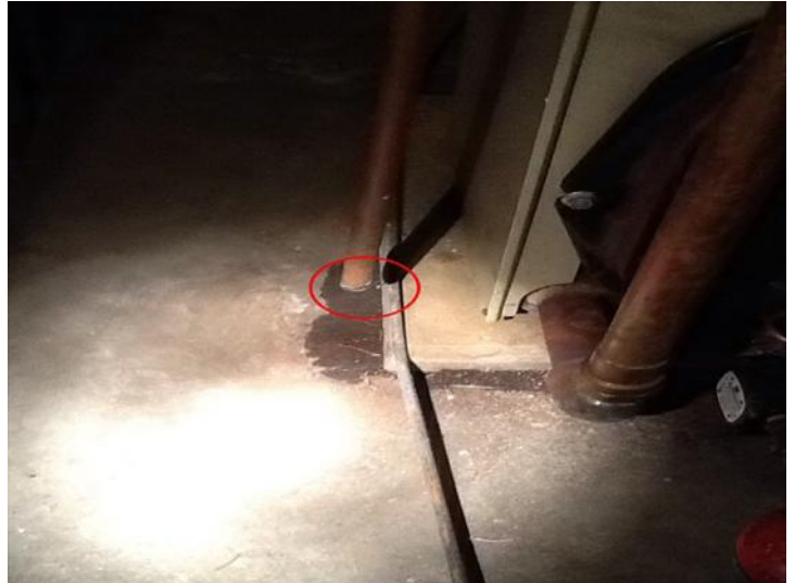
Repair leak at TPR valve and recommend servicing boiler system
