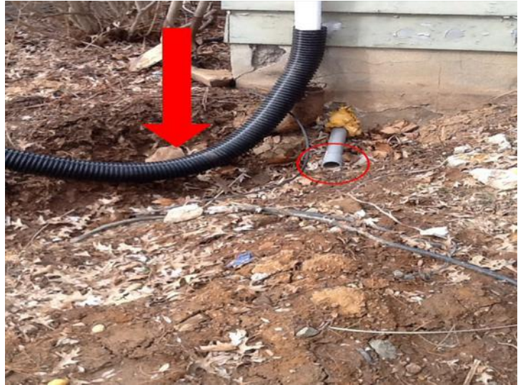
Correct grading so soil slopes from structure to direct water away and backfill SW areas, seller stated it is from a past underground electric service that has been removed. Cap opened conduit at wall.
