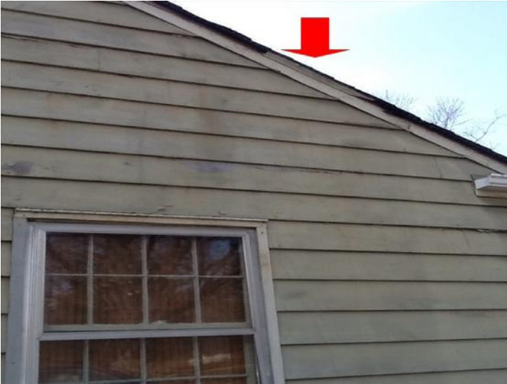
Trim damage/missing at East fascia
