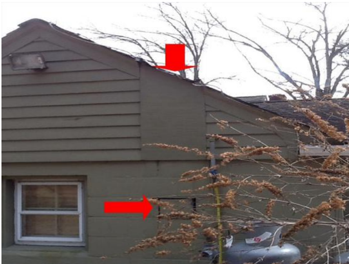
It appears there was a chimney at rear wall at one time and has been removed - patch roof shingles and block wall as needed.
