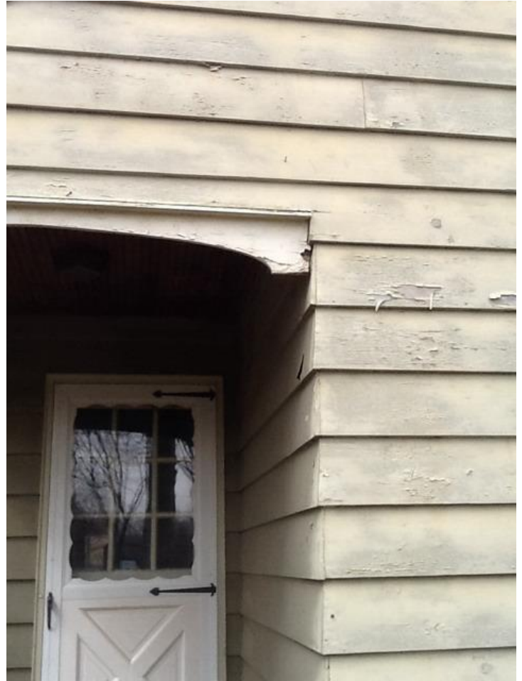
Trim has moisture damage and is in need of repair or replacement. Siding and trim need painting.
