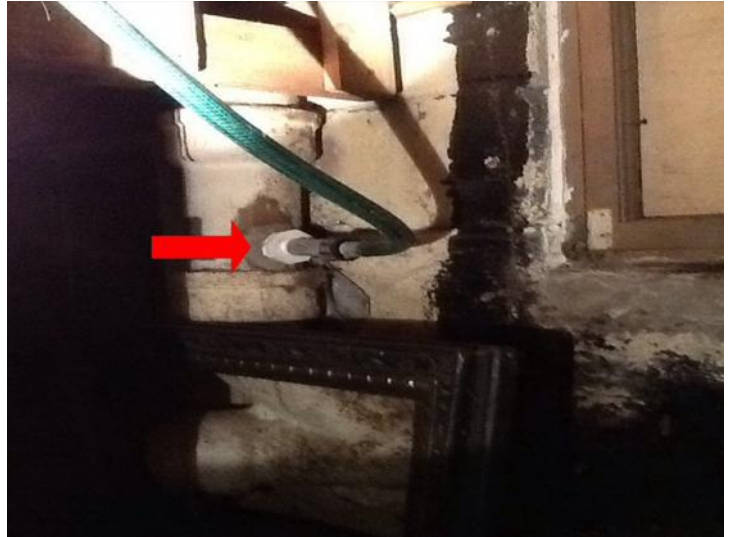
Sump pump ties into main drain line in basement - remove, cap and drain to exterior
