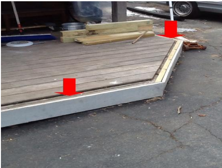
Install missing trim at deck perimeter
