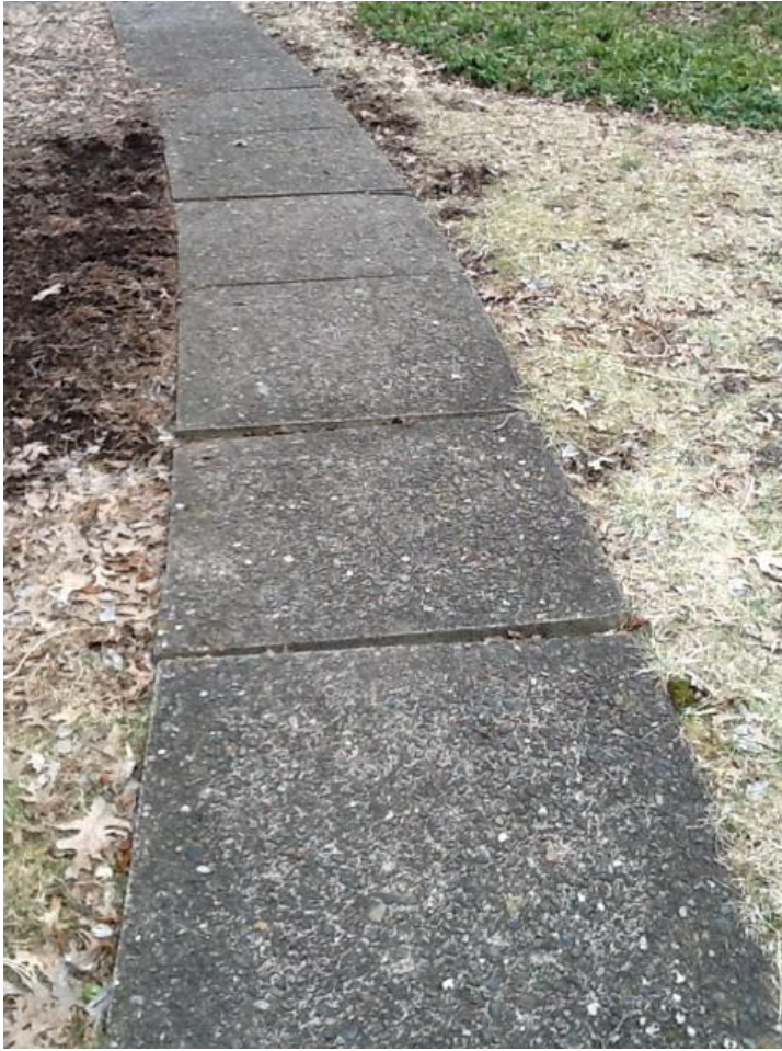
Uneven sidewalks, could be a tripping hazard, repair and/or replace as needed.
