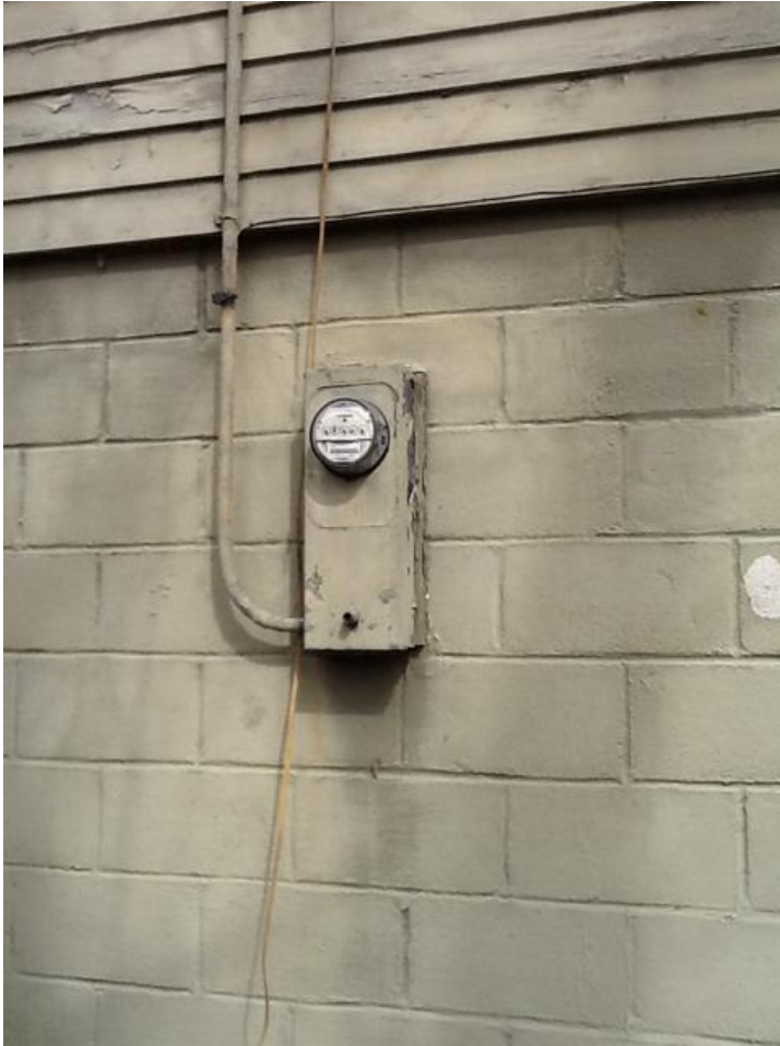
Electric service/meter
