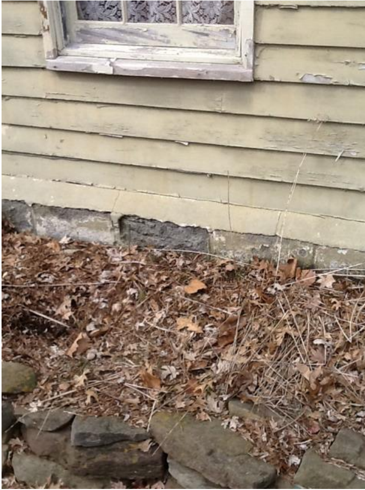
Surface deterioration to areas of exterior block foundation and walls - patch as needed
